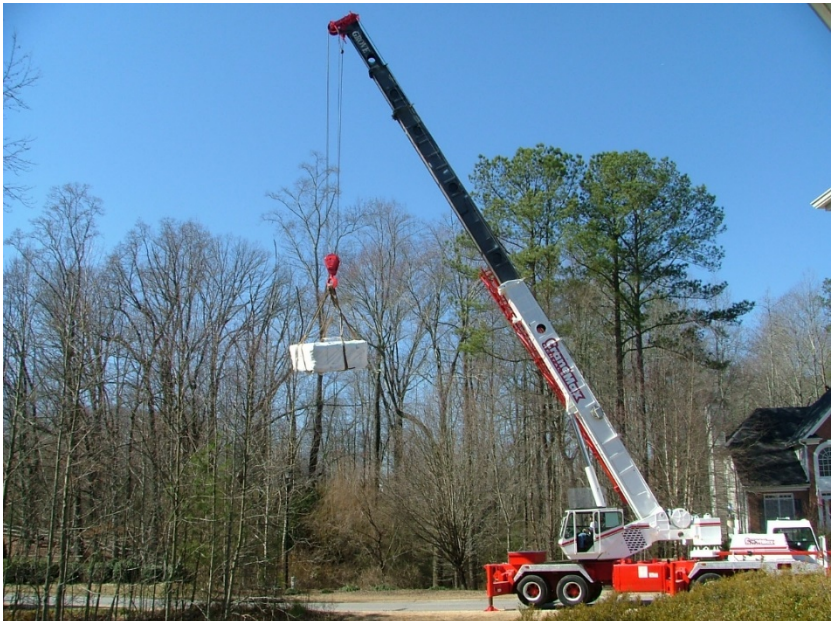
Figure 3 – A Crane is a Common Delivery Arrangement for Swim Spas
