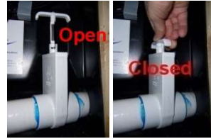
Figure 16 - Valve Open/Closed
